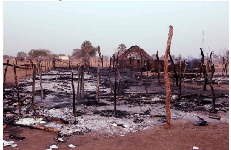
The village school which recently burnt
