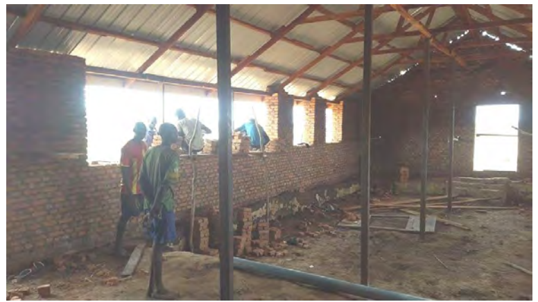
Reconstruction of the inside of the building in progress
