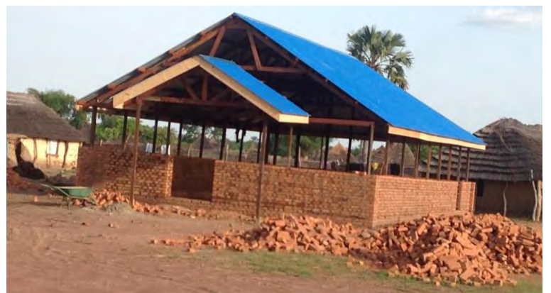
The outside of the building during reconstruction
